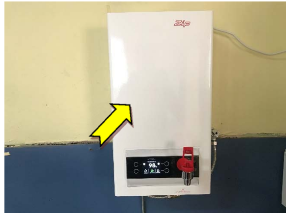
Photo 2. Interior, kitchen, hot water heater – suspected SMF internal insulation.
