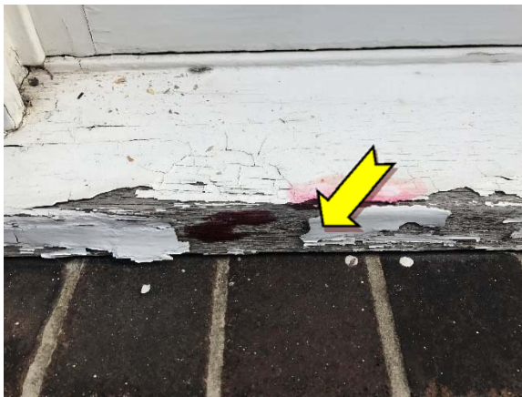
Photo 3. Exterior, throughout, window frames – suspected lead-containing white upper paint system.
